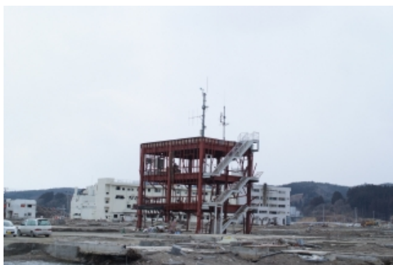
Minami-sanriku Town Hall (April 14, 2012)
