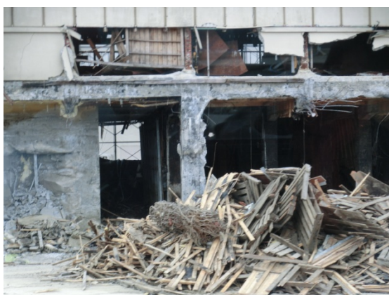
Kesen-numa Port facility (April 14, 2012)
